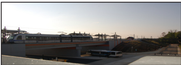
(LYNX's South Boulevard/I485 station, with bus transfer and parking deck right)
