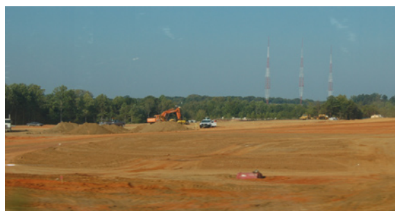
(Parcel under development along the LYNX line, near Arrowood)
