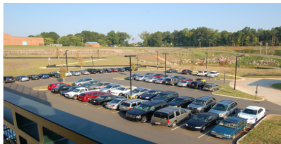
(Paved overflow lot, I485/South Boulevard)
