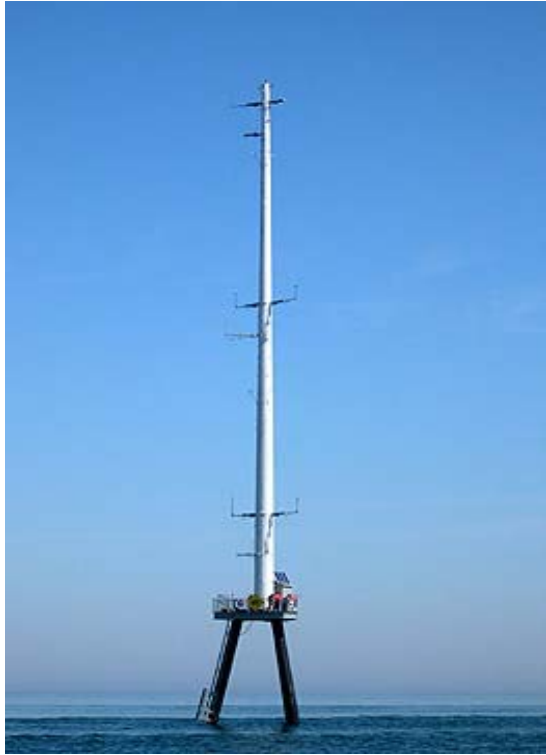
Figure 3-5 Example of Monopole-mast Meteorological Tower
